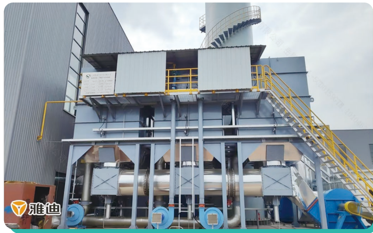
RTO treatment equipment in the production base
