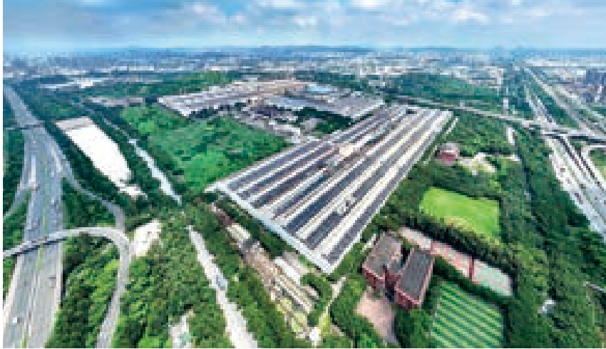
Distributed PV power station in Guangzhou, Guangdong province
