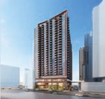
Bailey Street/Wing Kwong Street Development Project, To Kwa Wan, Hong Kong (artist's impression)
