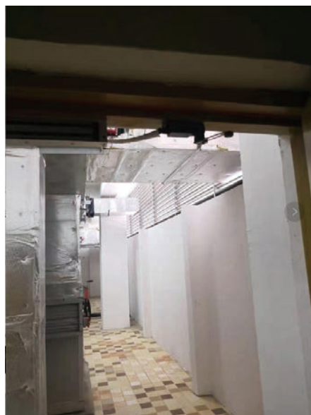
(Install on-line switches for all equipment rooms, light on the door, and turn off the door) (對所有設備機房安裝行程開關，開門燈亮，關門燈滅)
