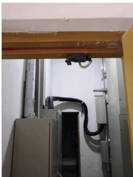
(Install on-line switches for all equipment rooms, light on the door, and turn off the door) (對所有設備機房安裝行程開關，開門燈亮，關門燈滅)
