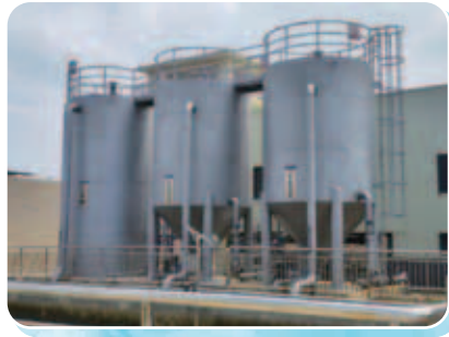
Equipment Applied with Cyclone Granulation Thickening Technology
