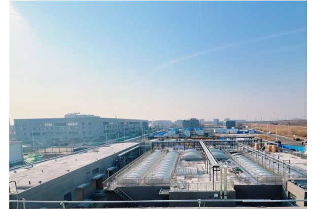
The Sewage Station Under Construction
