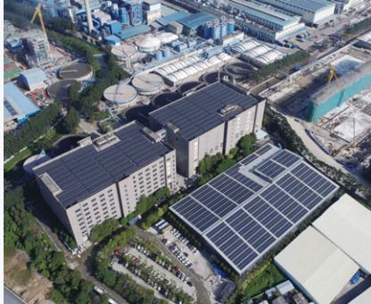
Rooftop Solar Power Project 屋頂光伏發電
