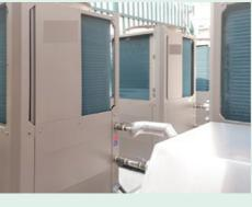
In addition to energy innovation and optimization in production regions, the Group also focuses on energy efficiency in non-production regions. In 2023, we pilot the Air Energy Water Heater for dormitories, heating the water through the valley electricity. Through the pilot, found that the consumption of air energy water heaters is more energy efficient than traditional outsourced steam heating, saving about 30% of energy use compared to the previous period.
