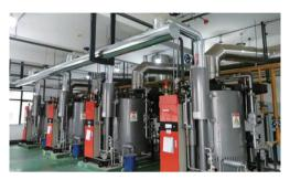
Low-nitrogen burners used for the gas-fired boilers in Beijing plant
