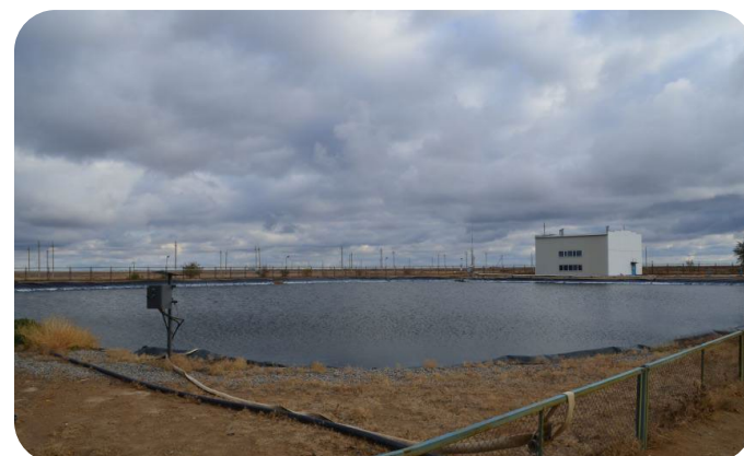
Ortalyk's wastewater treatment plant
