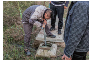
Shutting off Water Pipe Valves
