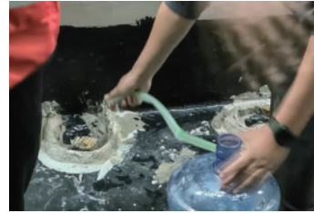
Testing Drainage System
