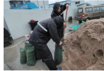
Making Flood Control Sandbags
