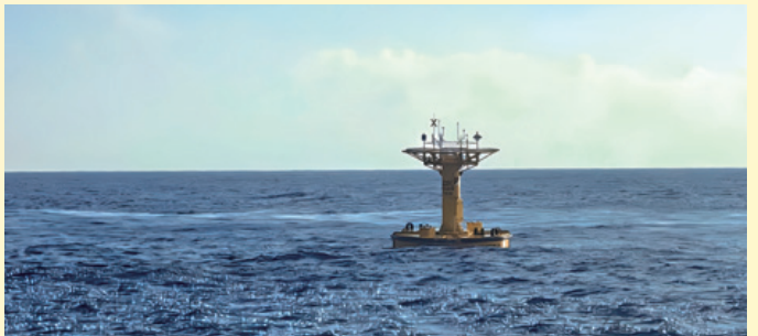
Anemometer tower of the Yangjiang Sanshandao's Fourth Offshore Wind Power Project
