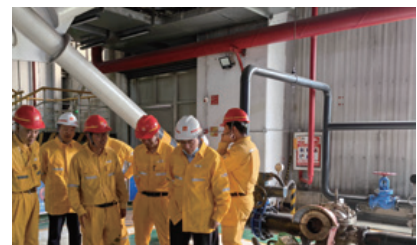
Safety inspection of unit maintenance site in Heze Company
