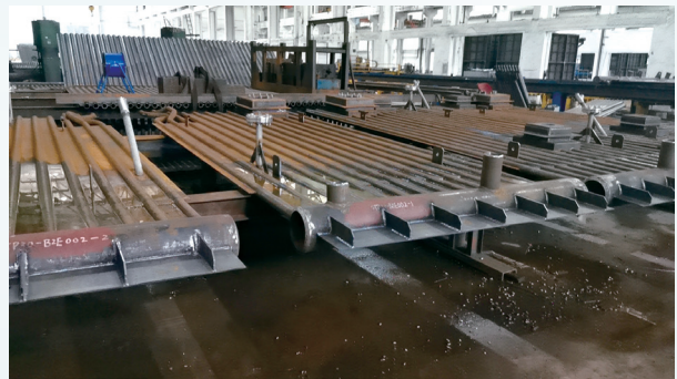
Installing Four Screens on Left and Right Walls of the Flue
