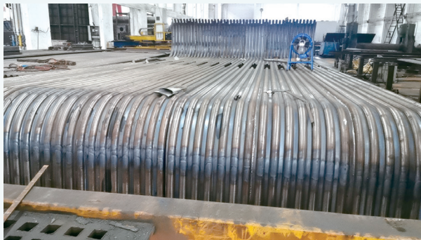
Installation of Water Cooling Wall on Site
