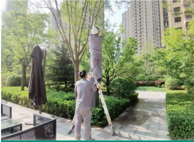
Replacing 200W light bulbs with 50W ones
