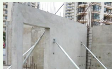
Prefabricated wall panels
