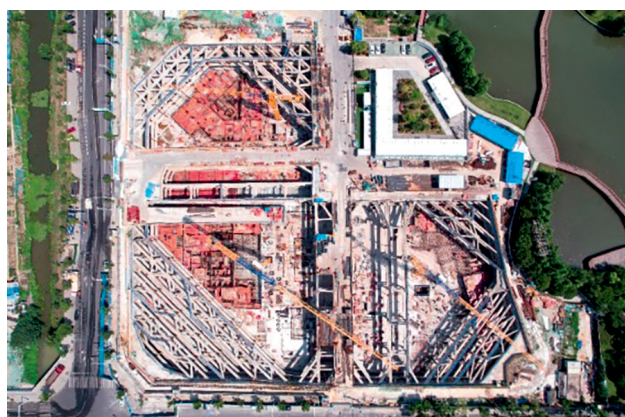
Concrete Bracing Pit Support
