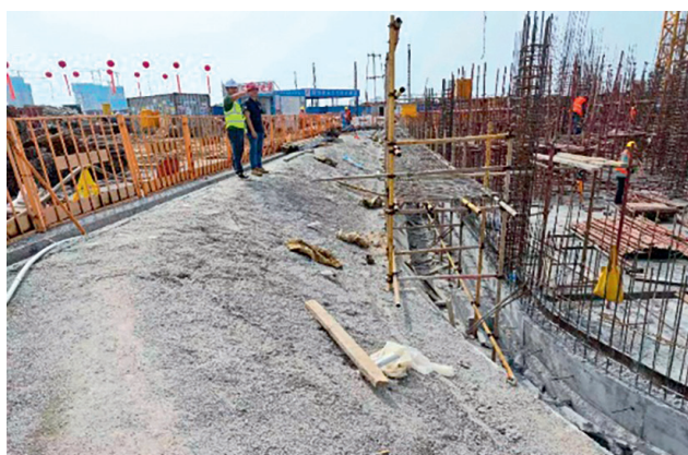
Anchoring and Shotcreting Pit Support
