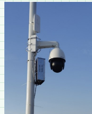
Surveillance camera at the edge of the excavation
