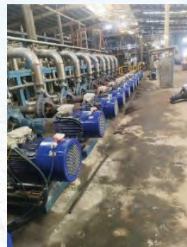
Replacement of high-efficiency rare earth permanent magnet motors for powder cyclones 粉旋流器更換高效稀土永磁電機
