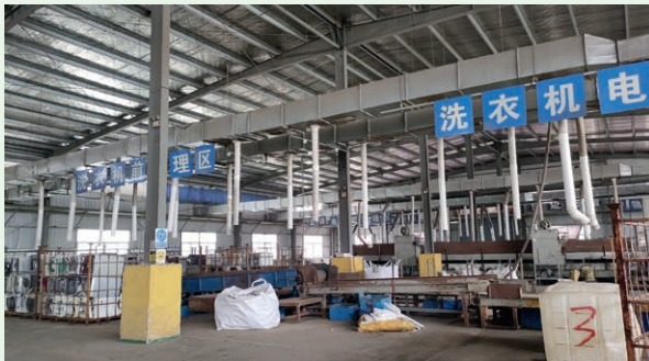
Cooling duct lengthened
