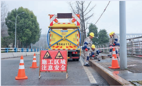
Conducting road maintenance
