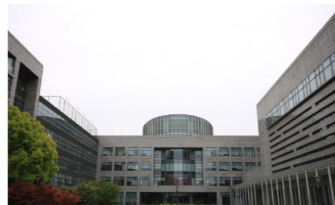
Shanghai Data Center
