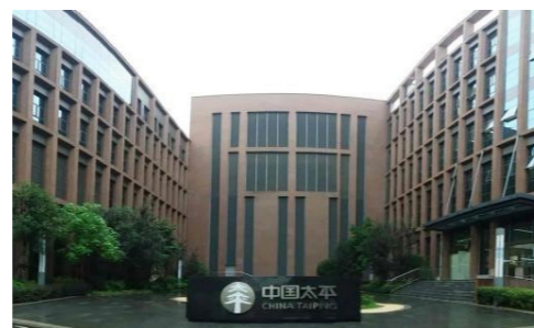
Wuhan Data Center
