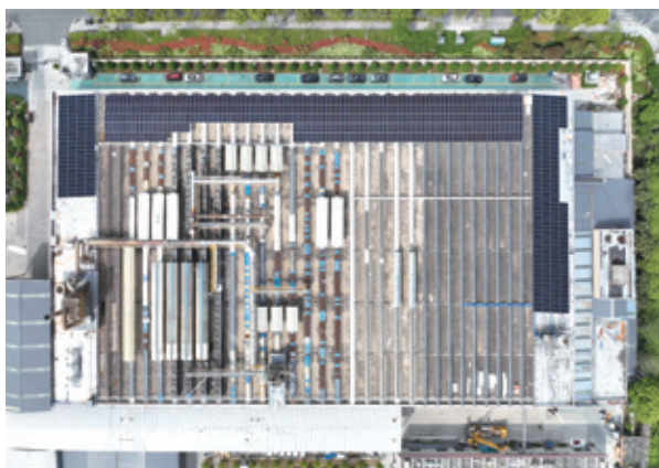
Current rooftop of the factory area
