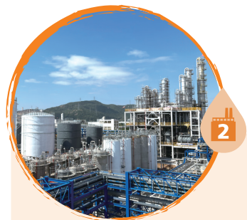
位於廣東珠海的溶劑廠房 The solvents plant in Zhuhai, Guangdong
