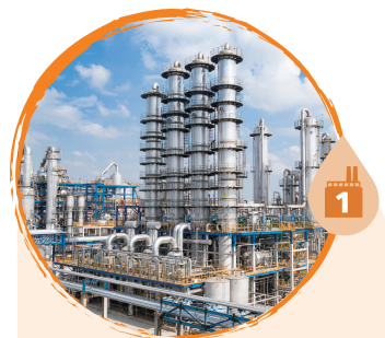
位於江蘇泰興的溶劑廠房 The solvents plant in Taixing, Jiangsu
