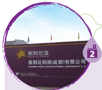
位於四川成都的塗料廠房 The coatings plant in Chengdu, Sichuan
