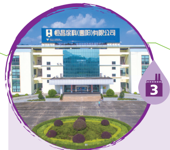
位於廣東惠州的塗料廠房 The coatings plant in Huizhou, Guangdong
