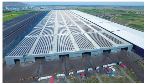
Tuyou Photovoltaic Power Plant + Factory Roof
