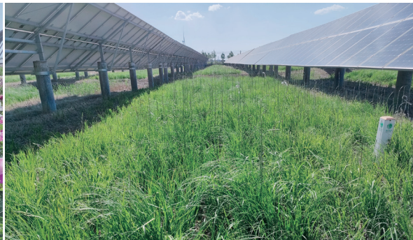
Tangshan Photovoltaic Power Plant + Rhizoma Anemarrhenae 唐山光伏電站+知母
