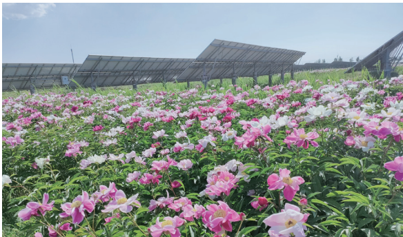
Tangshan Photovoltaic Power Plant + Peonies 唐山光伏電站+牡丹
