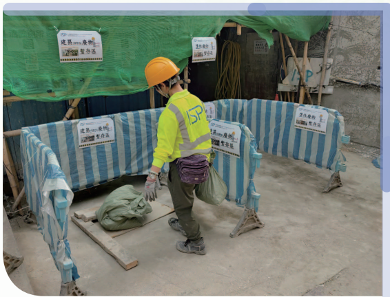
Separation of inert and non-inert waste at the construction site 建築工地上惰性和非惰性廢物的分類
