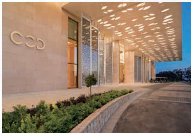
City of Dreams Mediterranean brings the Group’s award-winning standards of entertainment, leisure and innovation to Cyprus’ luxury hotel scene, marking a brand-new era for premium tourism in Cyprus.
