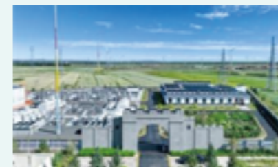
Views of Zhangjiakou-Beijing Renewable Energy Integration and Application Demonstration Project
