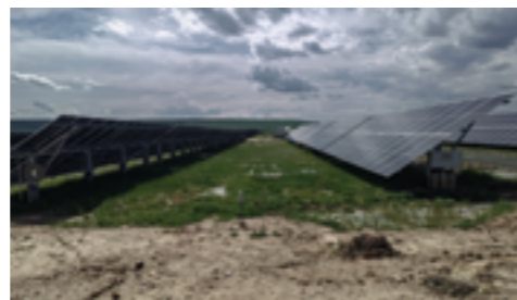
Photos of the Jixianghuaya Photovoltaic Project sand treatment
