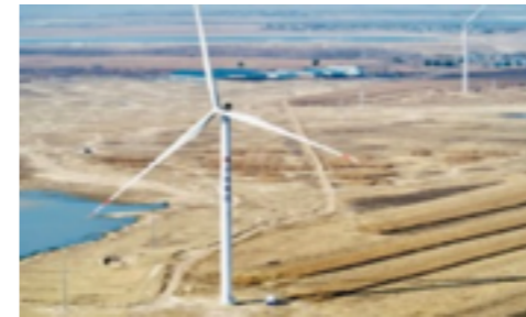
Daqing JINGNENG Wind Power Demonstration Project of Grid-Connected Electricity at Parity
