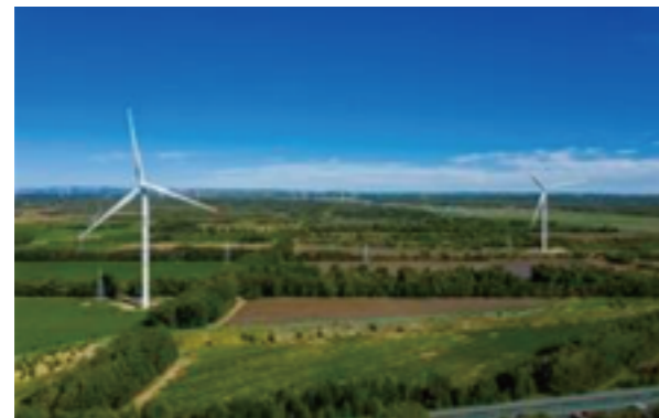
Zhangjiakou-Beijing Renewable Energy Integrated Application Demonstration Project
