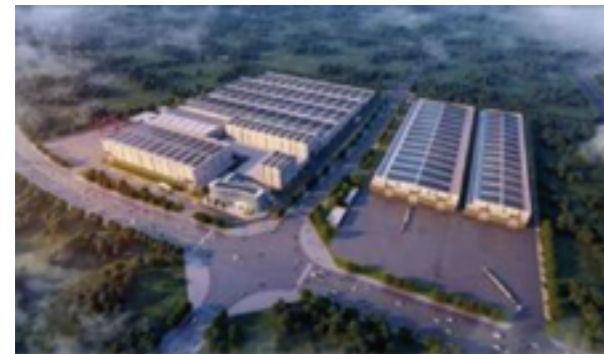
Image of the "Four Integration" Offshore Wind Power Equipment Manufacturing Industrial Park Project
