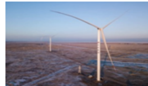
Daqing JINGNENG Wind Power Demonstration Project of Grid-Connected Electricity at Parity
