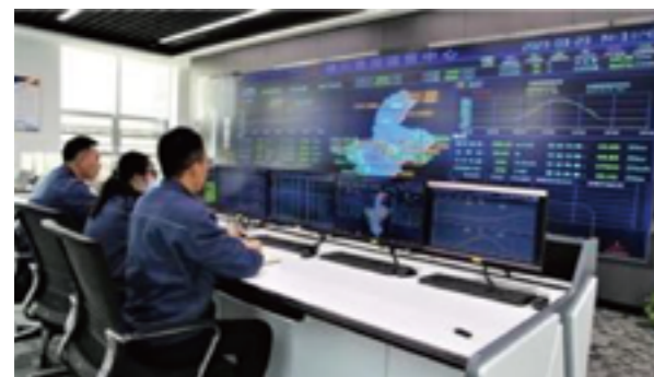
Northwest Branch Yinchuan Operation Control Center
