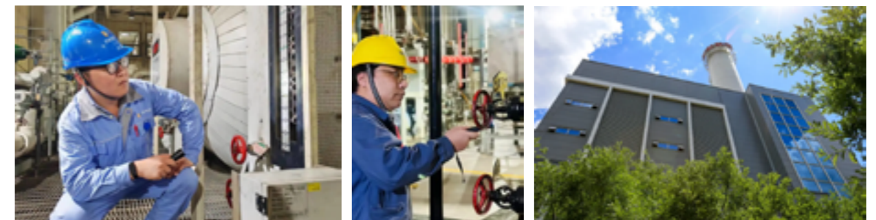
Jingyang Power guaranteed heating supply
