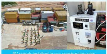
To enhance energy efficiency, the group has introduced solar energy systems in our construction sites to utilise solar energy as an alternative energy source. Currently, construction sites without electricity supply have strong reliance on diesel fuel generator for operations. Hence, the group is committed to exploring alternative energy sourcing options. By installing solar PV panels, we can reduce fuel consumption.
