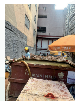
Wastewater treatment facilities in construction sites
