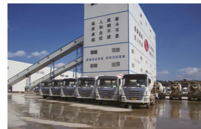
Noise control production system, belt enclosure
