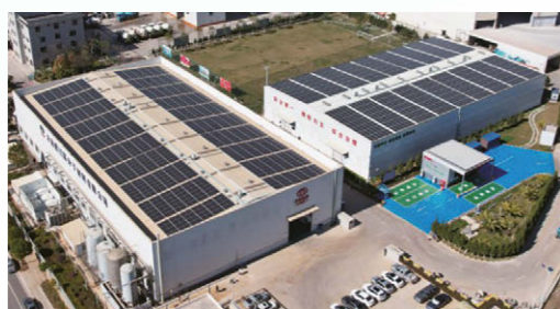
Rooftop distributed photovoltaic power station in Jingkai green production base- Phase I
