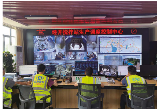
Remote central control for operating room of production system
