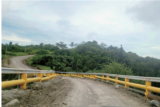
Downhill pavement reconditioning
