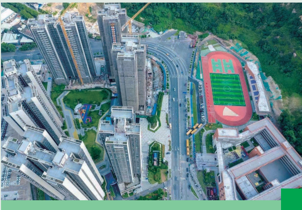
Phase III and Phase IV of the Renovated Area of the Bi Village Three Project
