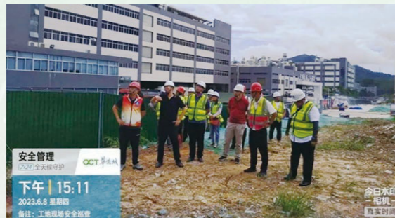
Safety inspection of the construction site of Entrepreneurship and Innovation Industrial Park
