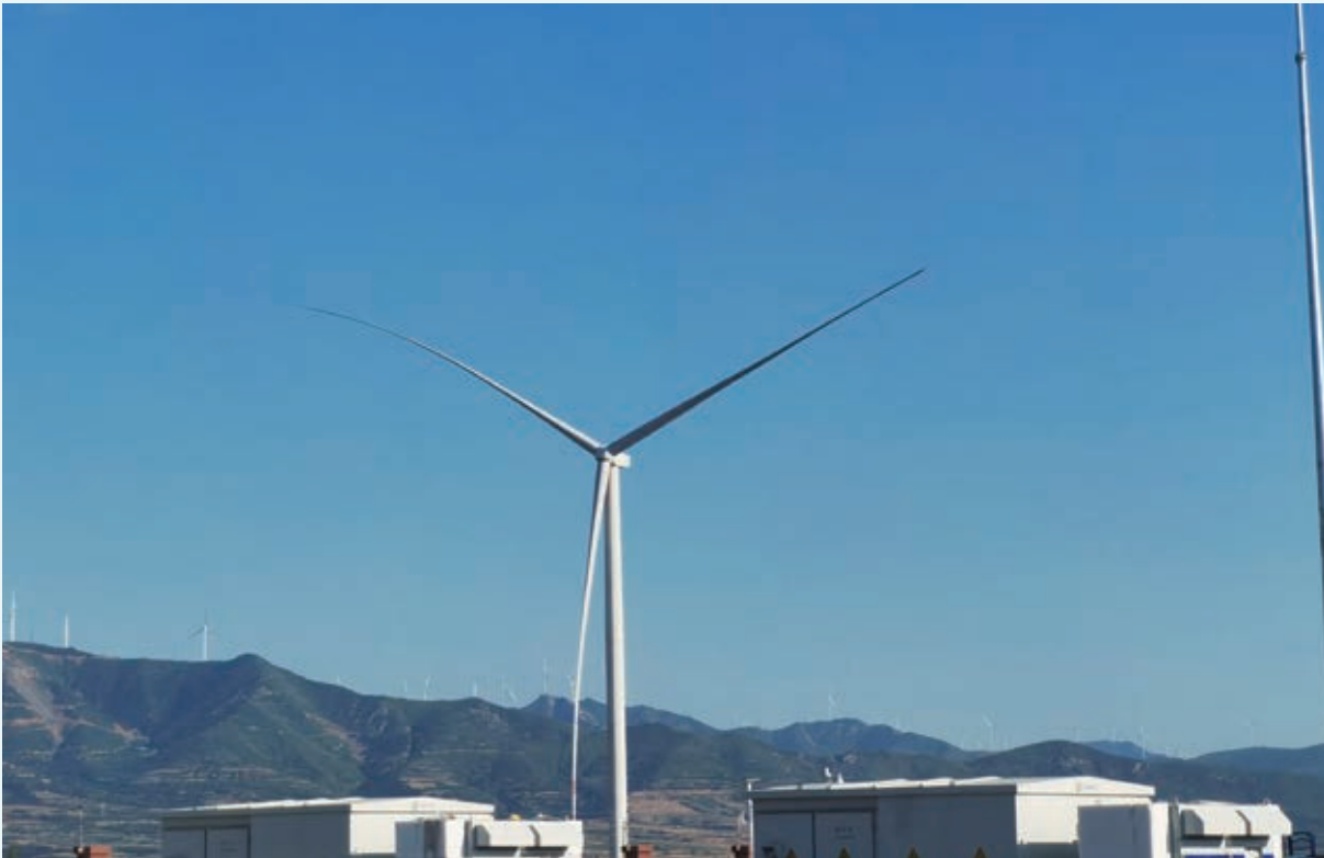
200MW Wind Power Direct Leasing Project in Wenxi County
