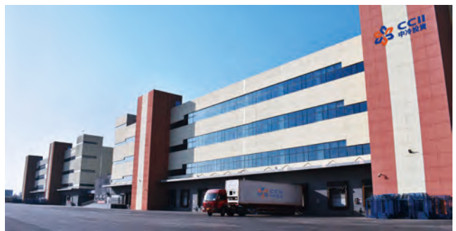
Tianjin Zhongyu Cold Chain Depot
