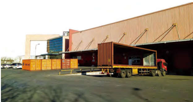
Tianjin Port Bonded Area International Logistics Center
