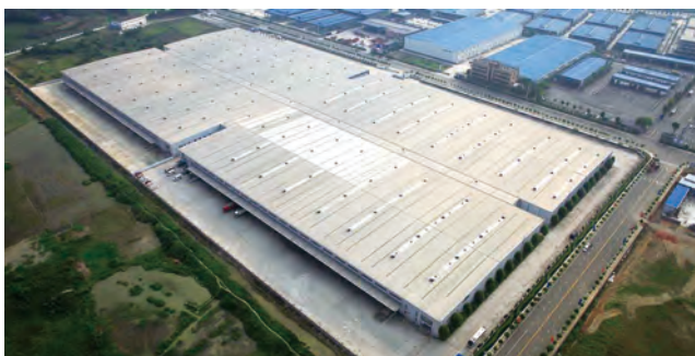
Meishan Xunda Hongtong E-Commerce Logistics Industrial Park
