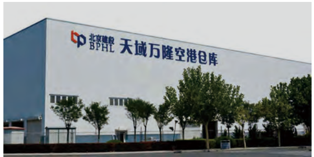
Transweath Airport Warehouse
