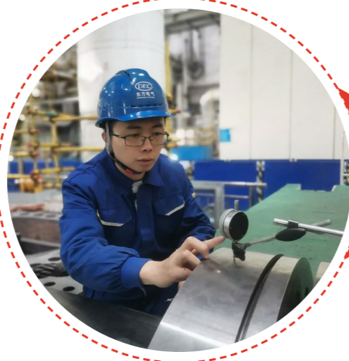
The power station service personnel of DEC Turbine was conducting lean maintenance of the generator set
