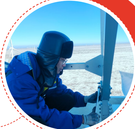
The team of DEC Wind Turbine Manufacturing Project checked the pre-tightening parts of the wind turbine blades at DEC Xing'an League Wind Power Base
