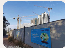
Spraying Facilities for Dust Reduction at Construction Sites
