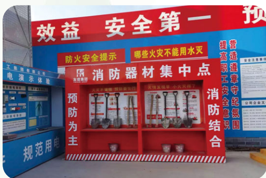
Fire Equipment Concentration Point
