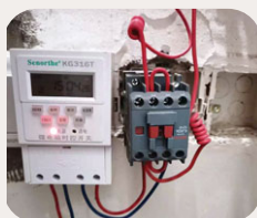
Installation of Time-controlled Switch
