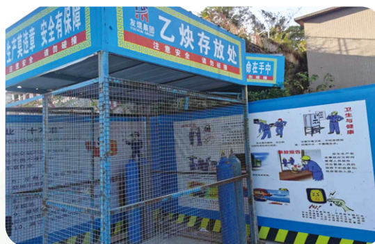
Storage Area for Flammable and Combustible Materials
