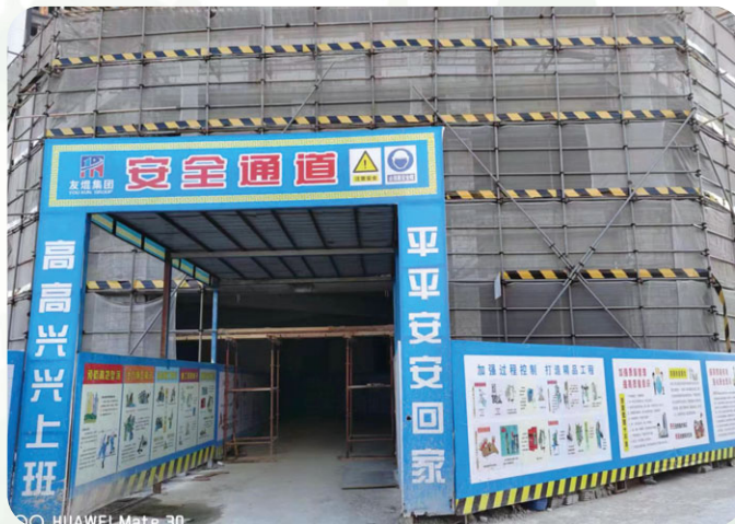
Construction Safe Passage
