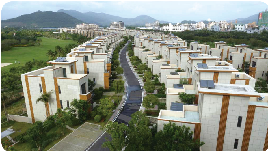
Solar Energy Systems Installed in the Clearwater Bay No. 3 in Hainan
