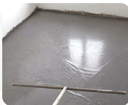
New Self-levelling Technology Application
