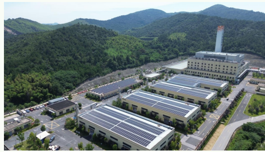
Huzhou Weineng Environmental Services Co., Ltd. 0.93 MW Photovoltaic Power Generation Project
