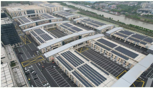
Huzhou Agricultural Products Wholesale and Distribution Center 2.72 MW Photovoltaic Power Generation Project
