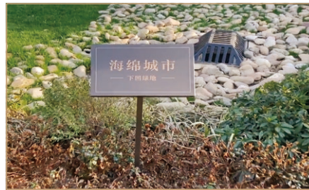
雨水花園、下凹式綠地、透水鋪裝示意圖 Illustrations of rainwater garden, sunken green space and permeable pavement
