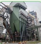
• The renovation from electric dust collection to bag dust collection machine for #1, #2, #3 kilns in Sichuan Ya Dong was completed, and the actual emission concentration of the dust is less than 5 mg/m³, which is lower than the local standard requirements.
