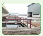
After sedimentation in the sedimentation tank, the wastewater is stored in the recovery tank and recycled for use in the factory
