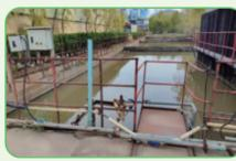
A rainwater and sewage sedimentation tank is arranged next to the raw material incoming road, and is used for flushing the raw material warehouse road
