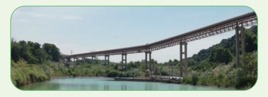
Fully enclosed corridor transportation project of Jiangxi Ya Dong After being crushed in the crushing workshop, the mine limestone is transported to the cement plant through the fully enclosed corridor, which not only saves energy and reduces dust pollution but also ensures efficiency and safety.
