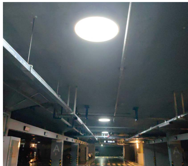
Tubular daylighting system
