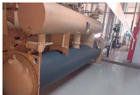
Freezer System Retrofit
