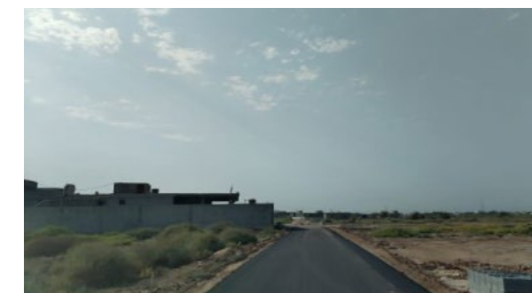
Construction Of General Roads in al Nashwa
