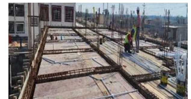
Construction of Al Zurajji Health Center
