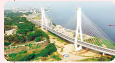
刚果（布）| 布拉柴沿河大道斜拉桥 Republic of the Congo|Brazzaville cable-stayed bridge along river
