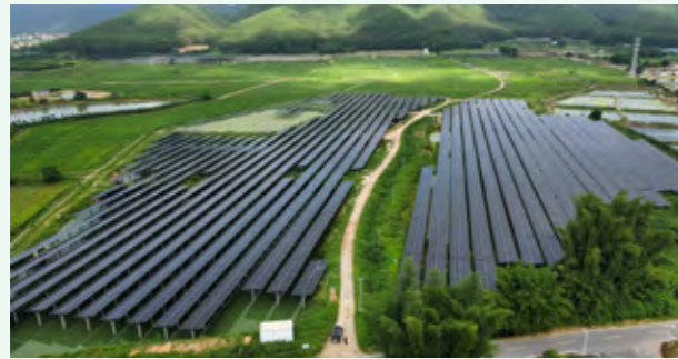
广东佛山水产养殖场“渔光互补”光伏电站项目 "Fishery-light Complementary" Photovoltaic Power Station Project of Guangdong Foshan Aquaculture Farm
