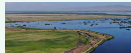
内蒙古乌梁素海山水林田湖草沙修复试点工程 Ulansuhai Mountain-Water-Forest-Farmland-Lake-Grassland-Desert Restoration Pilot Project in Inner Mongolia
