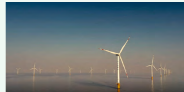
亚洲最大海上风电场——华能如东海上风电场 The Largest Offshore Wind Farm in Asia - Huaneng Rudong Offshore Wind Farm
