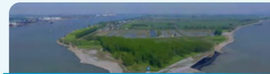
长江南京以下 12.5 米深水航道工程 Project of 12.5m Deep Water Channel of Nanjing-Taicang section of the Yangtze River Mainline:
