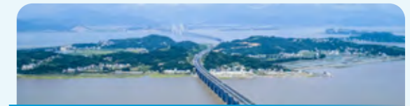
浙江省乐清湾大桥及接线工程 Yueqing Bay Bridge and Connection Project in Zhejiang Province:
