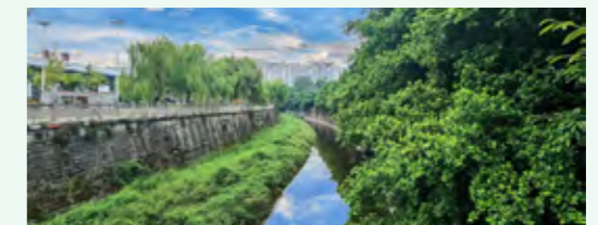
重庆万州区龙宝河综合治理工程（一期） Longbao River Comprehensive Treatment Project (Phase I), Wanzhou District, Chongqing
