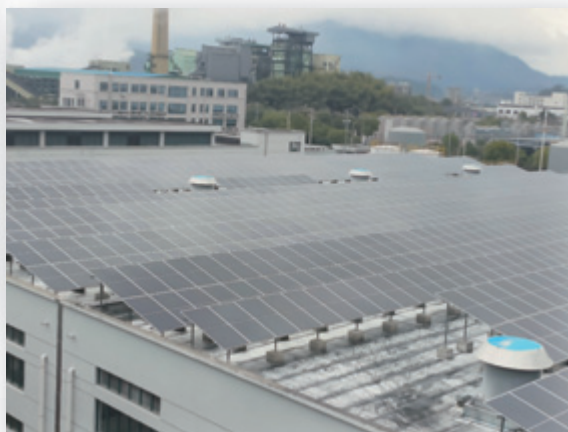
Install solar power generation equipment on the rooftop of factory
