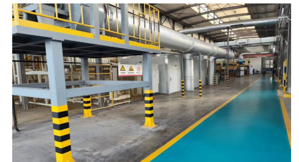
New project at the power spraying production line
