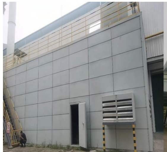
The noise control project of Ji'nan Drive Shaft Company for its coating line
