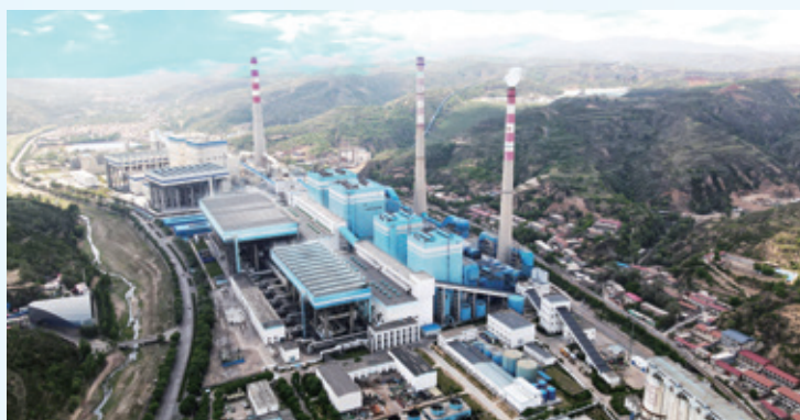
Taigu Heating Project — Substation of Energy Relay
