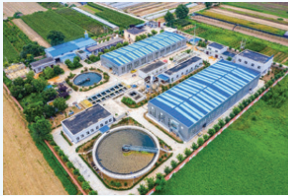
The Xia County Sewage Treatment Plant
