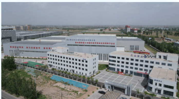
Main Structure of the Xiaohe Industrial Park Construction Waste Project
