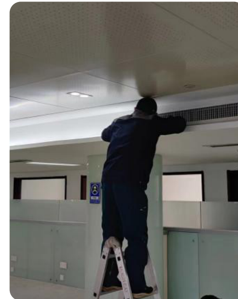
Replacement of energy-saving lighting fixtures by construction workers
