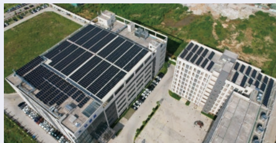
Roof-Mounted Photovoltaic Power Generation
