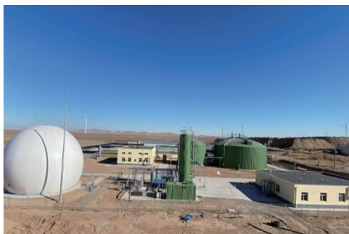
Chifeng Second Branch Biogas Station
