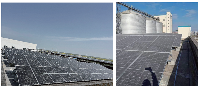
Newly built photovoltaic panels on the rooftops of the factories
