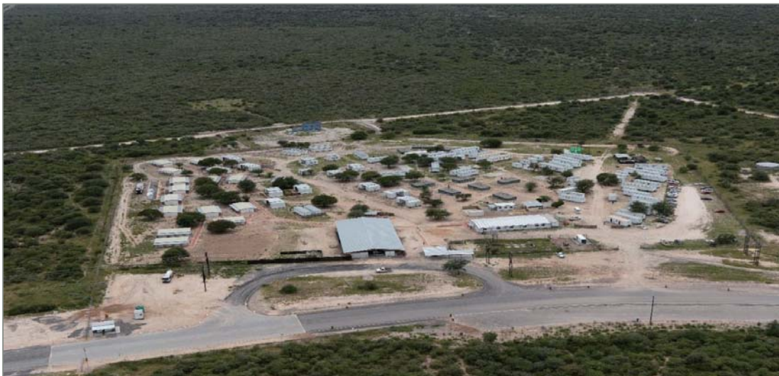
Figure 13-21 Tudika village – Boseto processing plant Source: KCM, 2023
