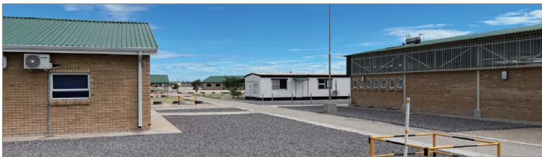
Figure 13-10 Zone 5 change-house and prefabricated training complex Source: ERM, 2023
