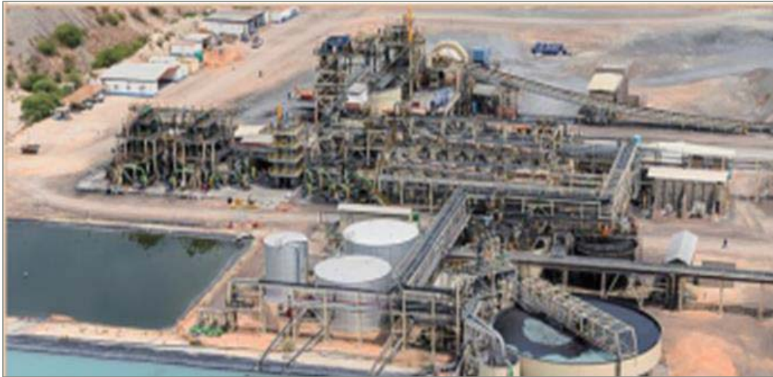
Figure 12-1 Aerial view of the Boseto processing plant Source: KCM presentation
