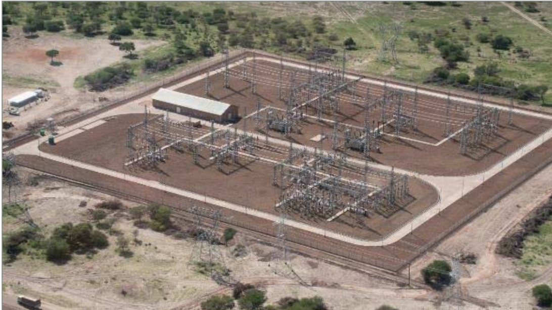
Figure 13-2 Newly constructed site infrastructure Source: KCM, 2023
