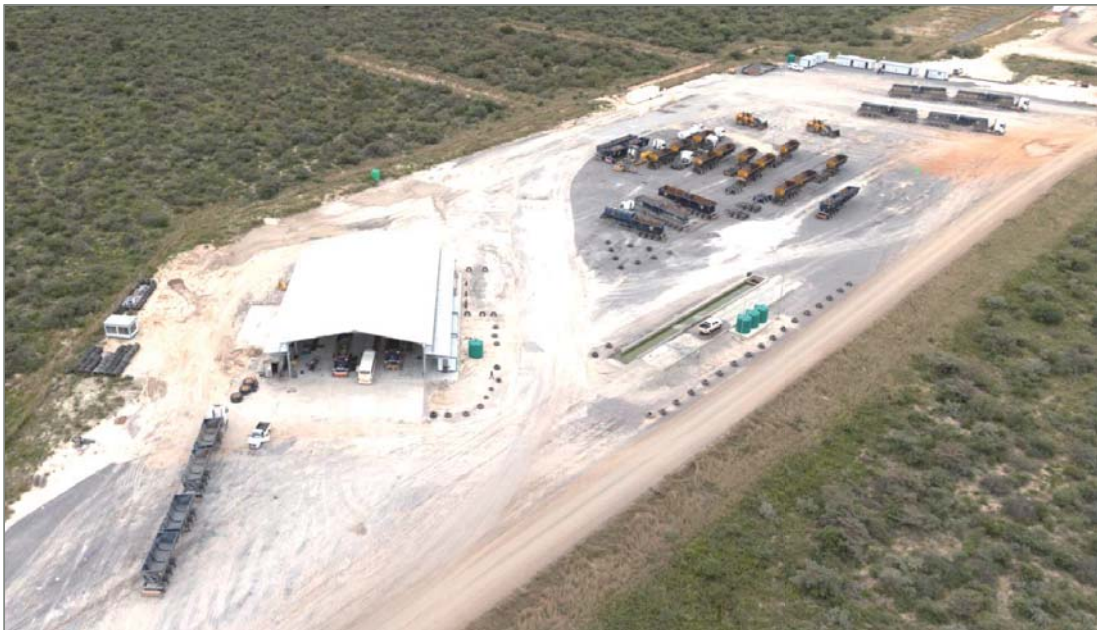
Figure 13-8 Ore haulage workshop and yard (Zone 5)
