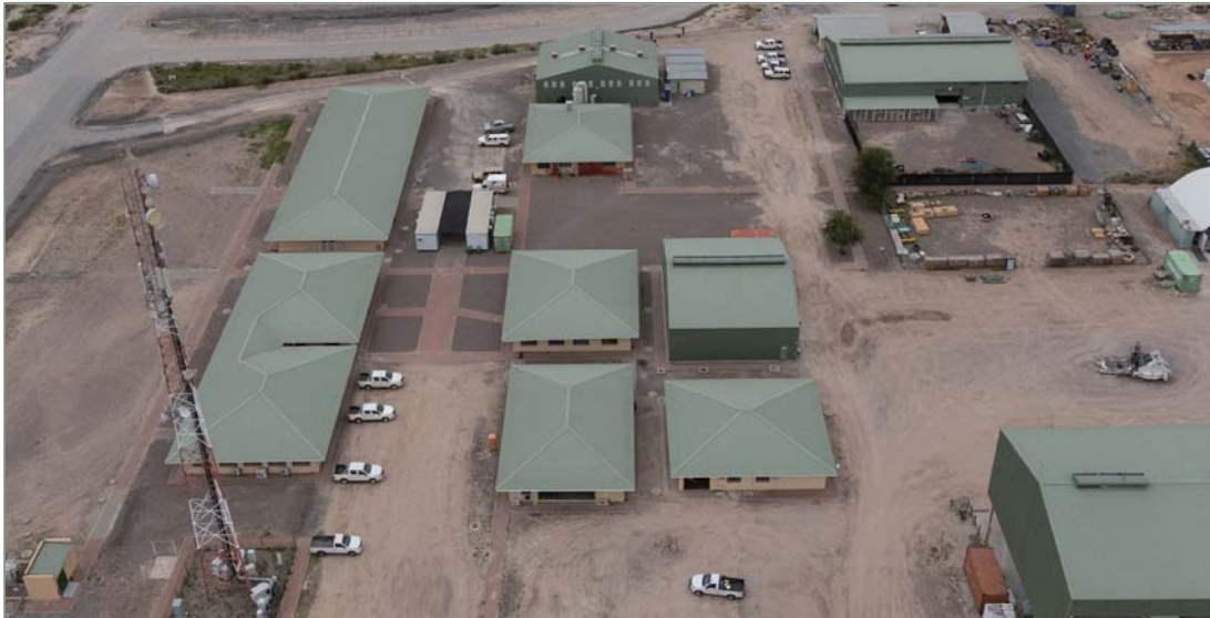
Figure 13-22 Cellular phone and radio communications tower Source: KCM, 2023
