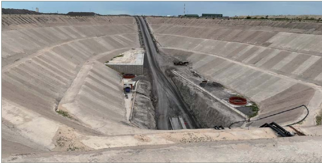
Figure 11-2 Zone 5 boxcut showing mine access and services
