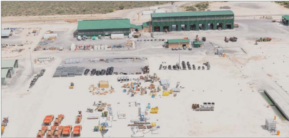
Figure 13-7 HME workshop and associated infrastructure at Zone 5
