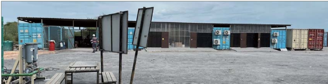
Figure 13-13 Miscellaneous storage – Boseto processing plant Source: ERM, 2023
