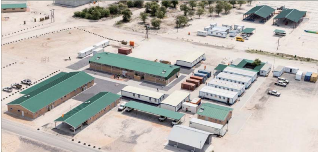
Figure 13-12 Aerial view of the Zone 5 office complex Source: KCM, 2023
