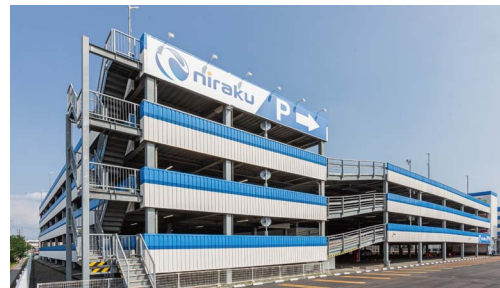
NIRAKU Koriyama Omachi hall's multi-story parking lot
