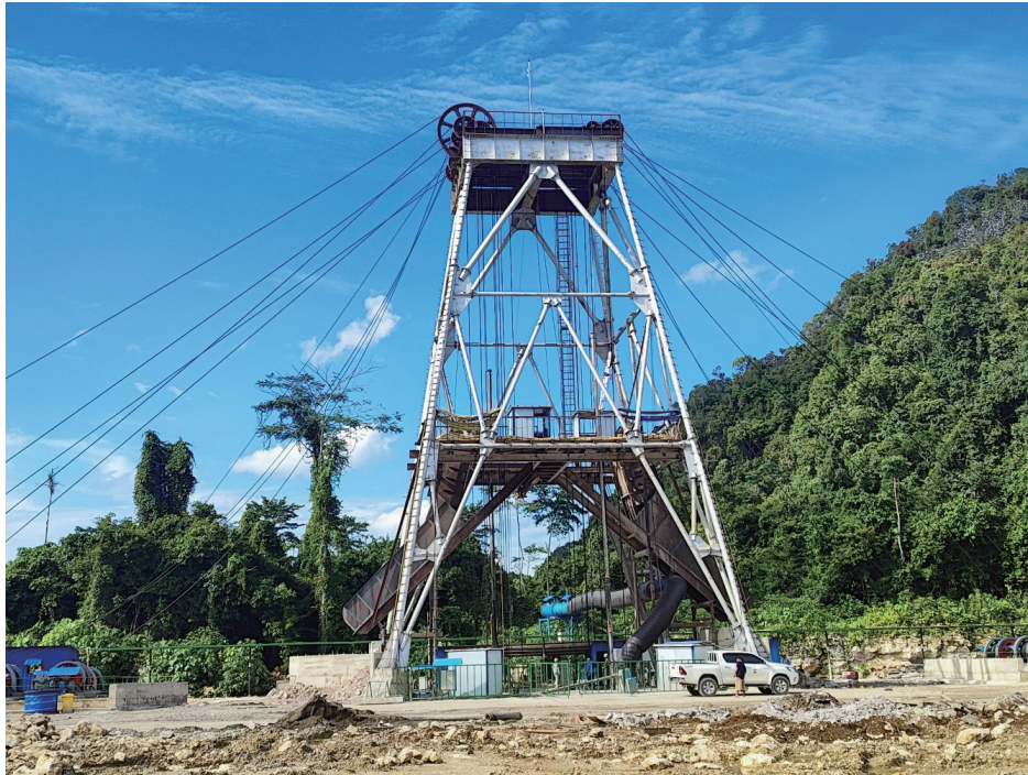
Figure 22: The Auxiliary Vertical Shaft of Qinfa Mine II
